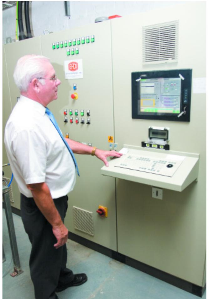
The upgraded graphical Windows based operator control station
